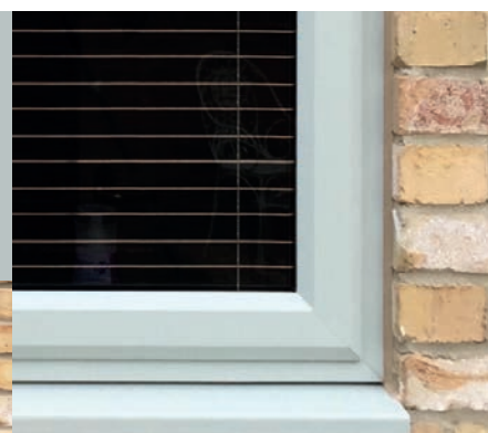
Welded joints on both outer frame and Rebated Sash
