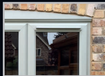
Trickle vent through a Rebated Sash
