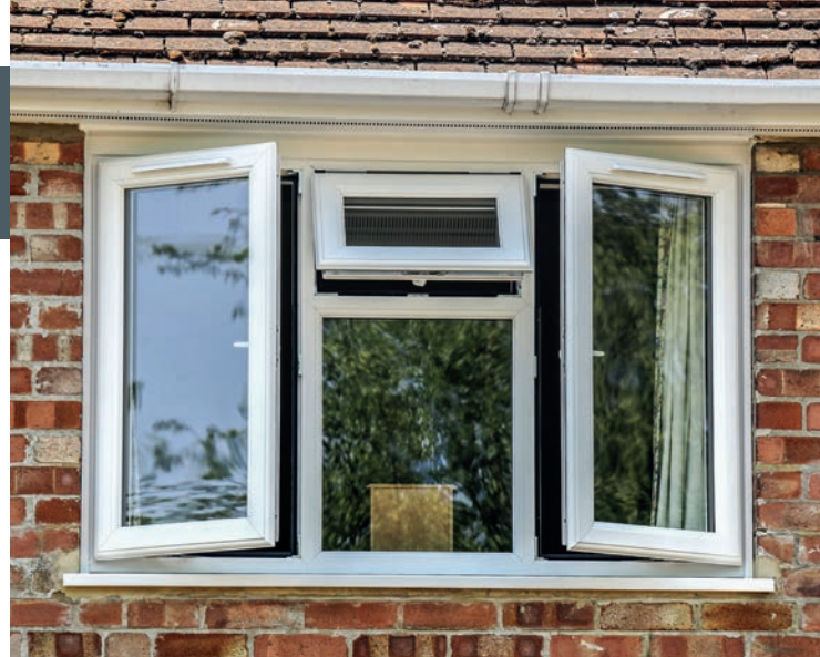
Trickle Vents installed through the window sashes
