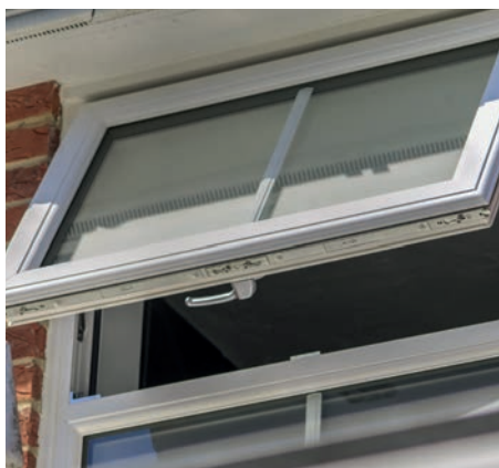
High Security Fire Escape / Easy Clean Hinges
